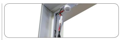
**Optional Jumper Cable:** For frames that are 8 feet or higher, use the jumper cable to put male and female connector together for the top edge lights.
