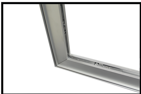
7. One corner finished! Repeat for the remaining three sides.
